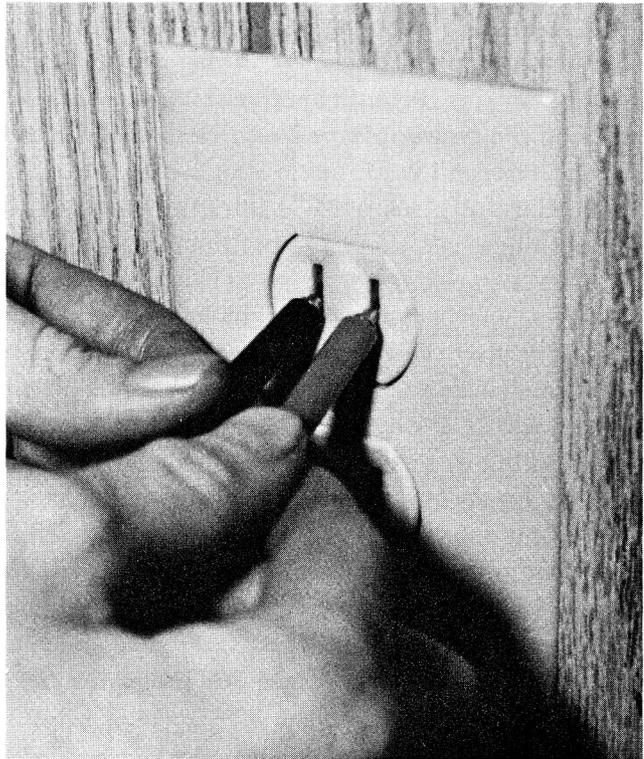
**FIG. 2-1** Using a meter to check for power.
