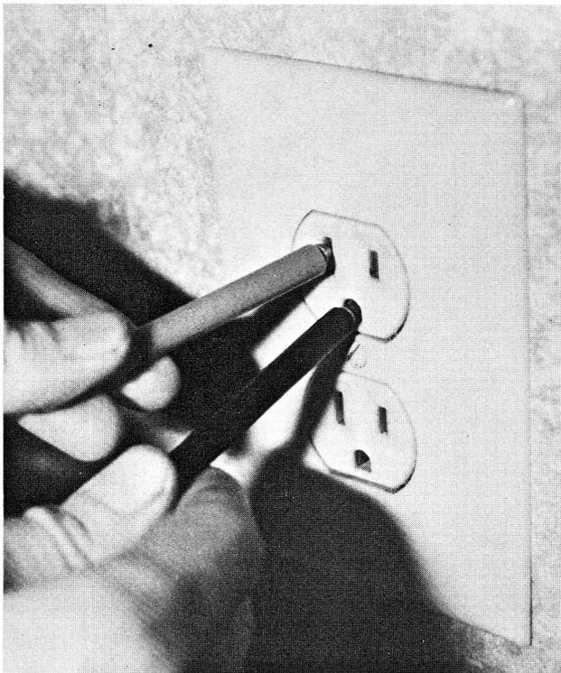
**FIG. 6-2** Checking an outlet with a meter.
